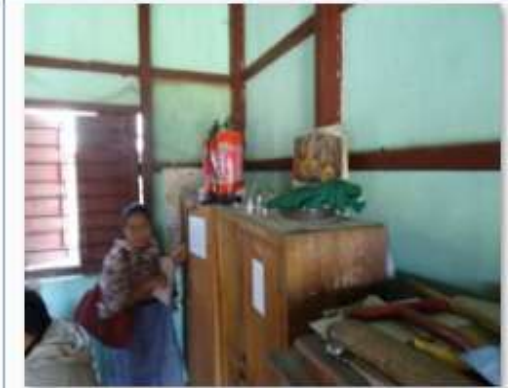
Fire extinguisher Bishnupur Awang Govt PS
