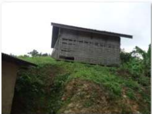
Kuccha Kitchen Shed Phoubut Primary School
