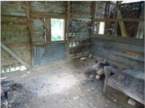
Tamah Govt PS Kitchen Shed
